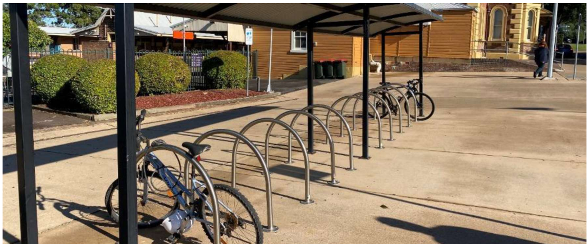
Figure 12 Bike racks located under a dedicated shelter at Maitland Station
